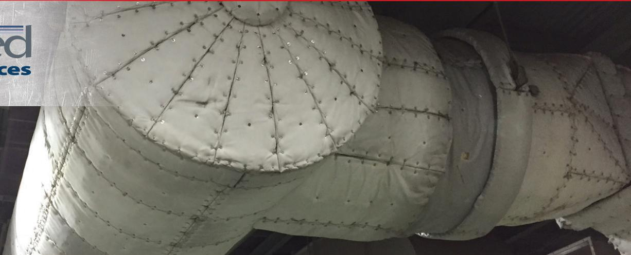
Through our vast experience in installing acoustic insulation panels and sound-absorbing jacketing, Advanced Industrial Services can provide noise control solutions ranging from industrial power plants to the smallest of construction projects.
